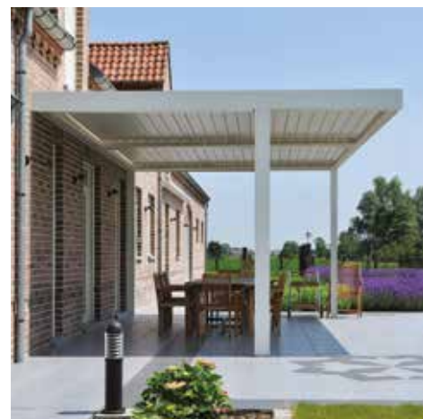
possibility of overhang up to 2m and up to max. 1/3 of the surface
